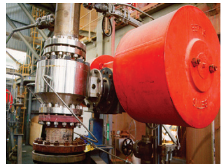
This 10-inch 300 Class discharge valve has been designed with purge ports per the customer's request.
