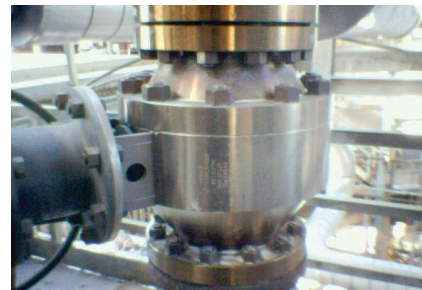
This CA-DRI 8-inch ASME 300 class valve handles catalyst at 1425° F (774° C). It is the major isolation valve between the third stage and fourth stage cyclone separator.
