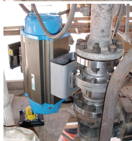
Installed between the lockhopper and lift engager at a major southwest refinery, these 3-inch ASME 300 class metal-seated isolation valves cycle at least three times an hour. These valves replaced another manufacturer's design that lasted only two months.
