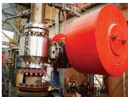
This 10-inch 300 class discharge valve has been designed with purge ports per the customer's request.
