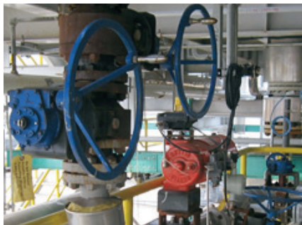
Twenty-five (25) CA-1AS 2-inch to 8-inch valves were chosen for this manufacturer of polycrystalline silicon materials and high-purity silicon products. Primary media was trichlorosilanes. All valves were oxygen cleaned in MOGAS' in-house cleanroom.
