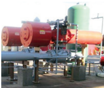
These 10-inch ASME 900 Class ESD valves installed in an ammonia plant have a stroke time of under 3 seconds.
