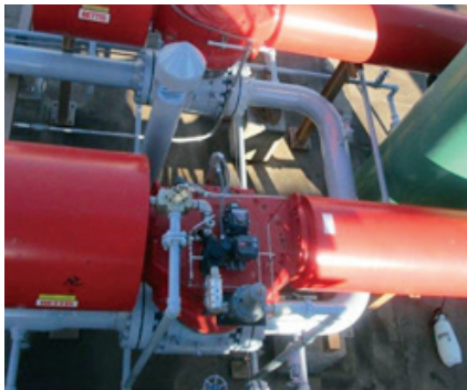
MOGAS CA-1AS valves reliably and safely operate to produce urea from ammonia and carbon dioxide.
