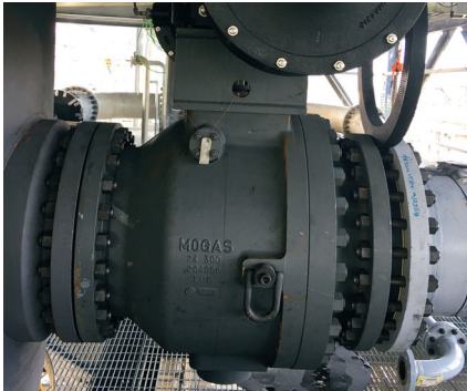
The installation of this 24-inch, ASME 300 Class T-Series trunnion was one of nearly 1800 valves for the start-up production of 1-butene.
