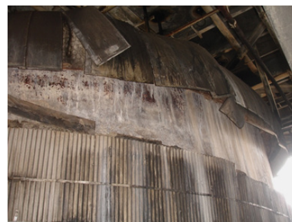
Leaking water from a competitor's valve caused damage to the coke drum's thermal insulation.
