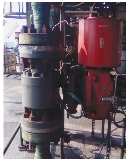
Above: One of several MOGAS 6-inch, ASME 2500 Class C-Series valve sits atop a coke drum in a South American refinery's cutting water application. This industry-proven valve is engineered specifically to perform in high erosion conditions.
