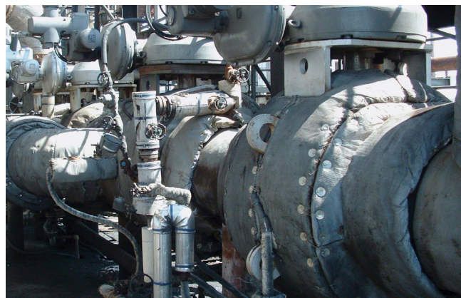
Four 20-in ASME 300 Class overhead vapor valves have been installed since 1991 at this refinery in Kansas, USA. After eight years of continuous service, less than 0.001 inch of the coating was worn away.
