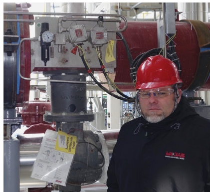
Above: One of several MOGAS 6-inch, ASME 2500 Class C-Series valve sits atop a coke drum in a South American refinery's cutting water application. This industry-proven valve is engineered specifically to perform in high erosion conditions.
