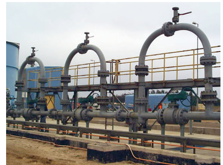
These 8-inch ASME 900 Class copper slurry valves have been cycling about 40 times per month against 1500 psi.
