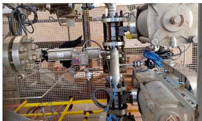
MOGAS primary and secondary acid injection valve designs, material selections and proprietary coatings have been proven effective for autoclave processes.
