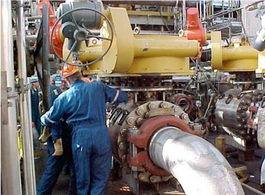
*Used in the upgrading of tar sands, this 18-inch, ASME 1500 Class isolation valve achieves positive isolation within 61 seconds. Previously used globe valves under the same conditions took hours, even shifts, to close.*
