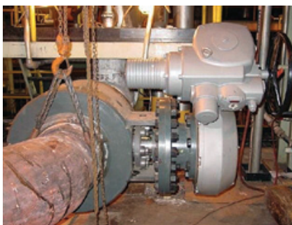
The new MOGAS metal seated ball valves were used in conjunction with a remaining gate valve as double-block and bleed.
