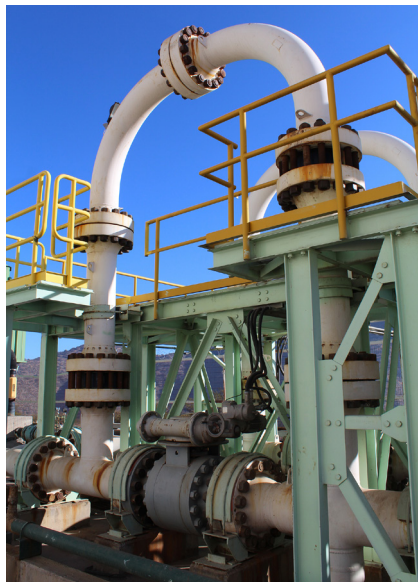
A MOGAS CA-1AS, 10-inch Class 1500 with electric actuation isolates the choke loop in a pressure letdown choke station for copper tailings in Chile.
