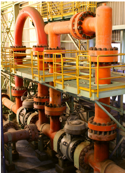
This MOGAS CA-1AS, 24-inch Class 900 with electric actuation isolates the choke loop in a pressure letdown choke station for copper slurry concentrate in Chile.
