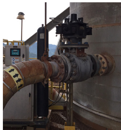
A MOGAS customized control valve with FlexStream technology cut depressurization time in half compared to its linear predecessor—all while staying well within strict noise, velocity and thermal-shock limits.
