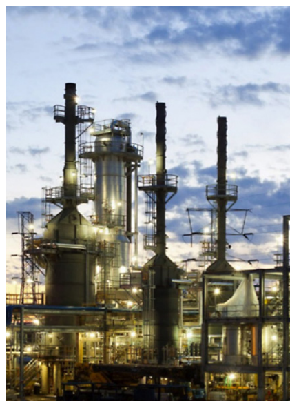
This modern re-refinery plant processes recycled oil through vacuum distillation and hydrotreating.
