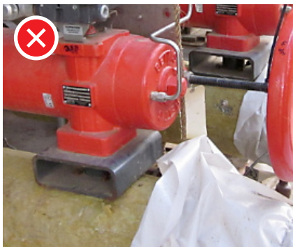
INCORRECT. Entire valve is covered.
