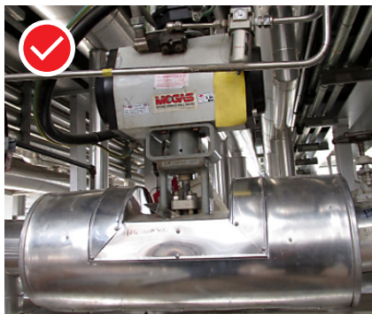
CORRECT. Packing box and stem exposed.
