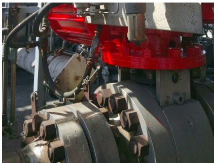
Located at a gasification project in China, this 8-inch 1500 ASME Class valve is for high-temperature oxygen service.
