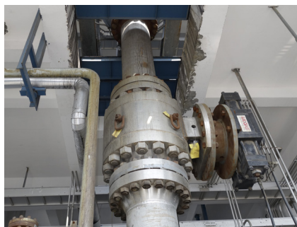
This 20-inch 900 ASME class valve with electrical-hydraulic actuator cycles every 30 minutes in operating conditions of 248° F at 1262 psig (120° C at 87 bar g.)
