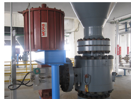
This 16-inch 900 ASME class valve was installed for slag water service, cycling every 30 minutes in operating conditions of 248° F at 943 psig (120° C at 65 bar g.)
