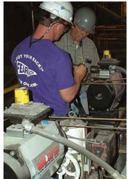
These four, 2-inch MOGAS ball valves are handling cold reheat isolation in a coal-fired plant.
