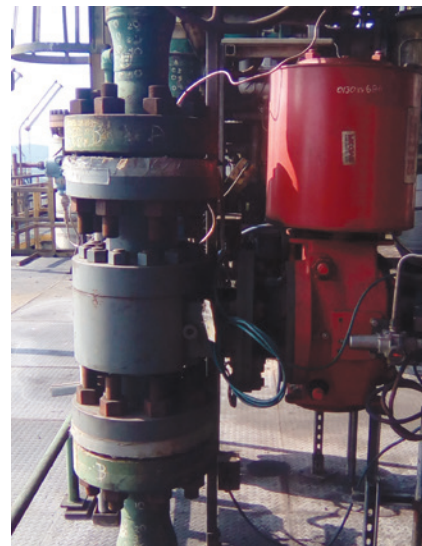
Above: One of several MOGAS 6-inch, ASME 2500 Class C-Series valve sits atop a coke drum in a South American refinery's water cutting application. This industry-proven valve is engineered specifically to perform in slurry and high erosion conditions.
