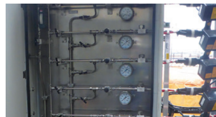
Multiple purge input lines can be combined into a shared cabinet based on geographical location of the purged valves in the plant.
